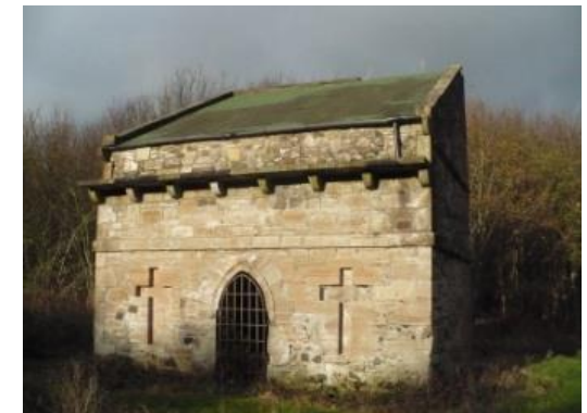
Dovecot, Eglinton Park, Kilwinning
